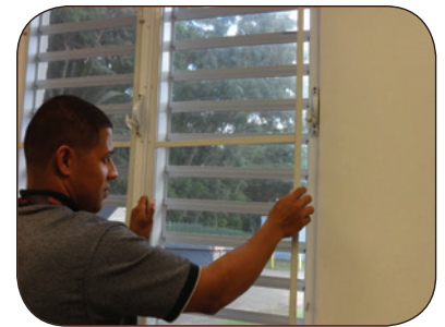
Install or repair window & door screens.
